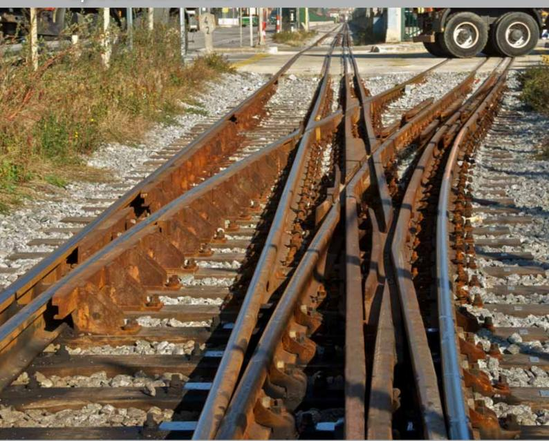
At Amurrio, we are specialists in the design, manufacture and installation of special turnouts for complex points. A good example of these is the coexistence of several track gauges in the same place, such as sea-ports.
